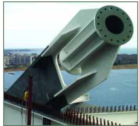
Above is a girder with an integral web connection. Below is a shark fin after installation of the bridge deck and connection to the cable.
