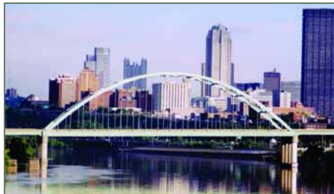
The bridge pictured above has a span-to-rise ratio of 4, while the one below has a span-to-rise ratio of 6.
