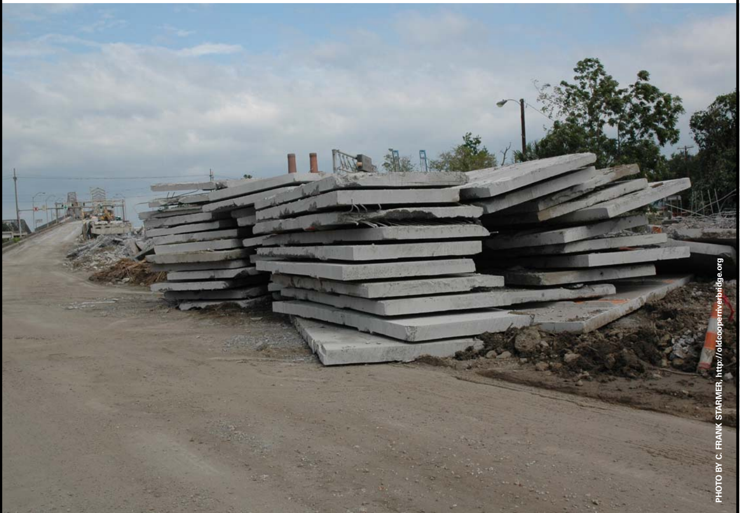
By the Fall of 2005, CCB operators had cut 60,000 lineal feet of 8-inch-thick concrete.
