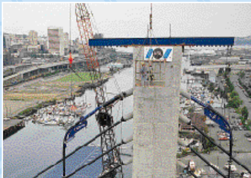
▲ installation of the stays
