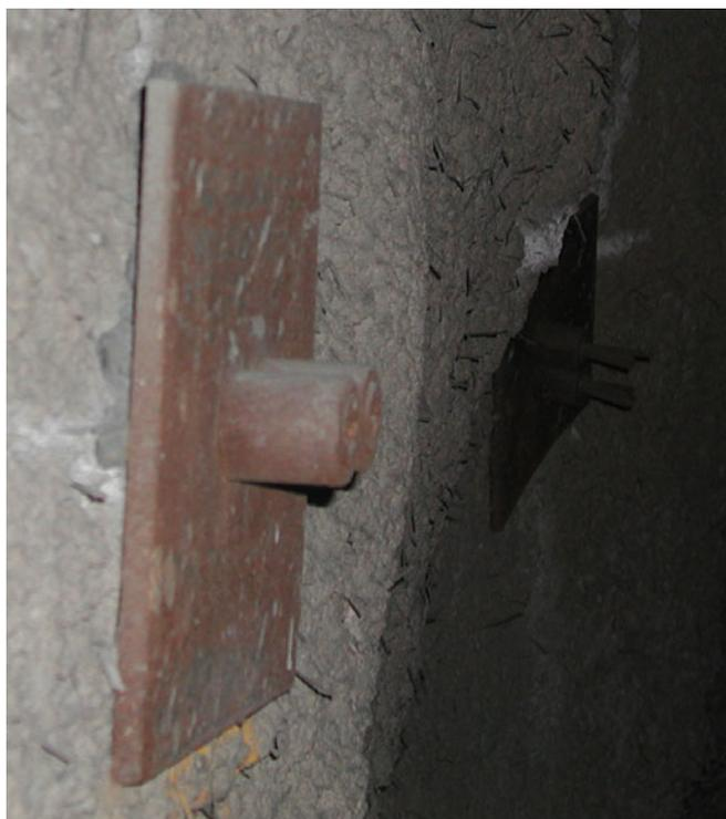
Figure 1: Anchors with strand receded compared with original position observed in a WA mine.
